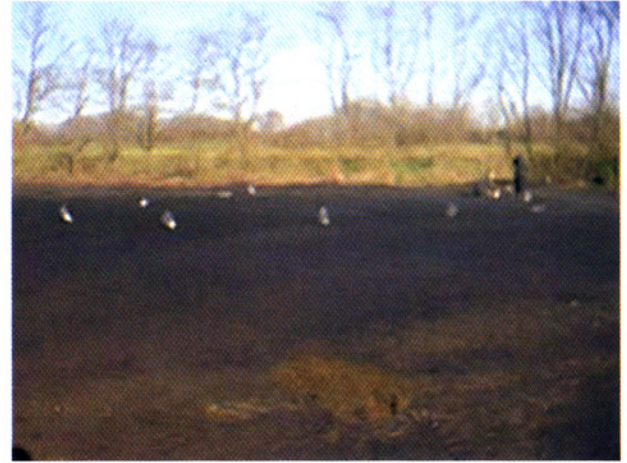
Prior to dredging, samples were taken. In the future, mapping the settling pond may provide a more consistent feed.
