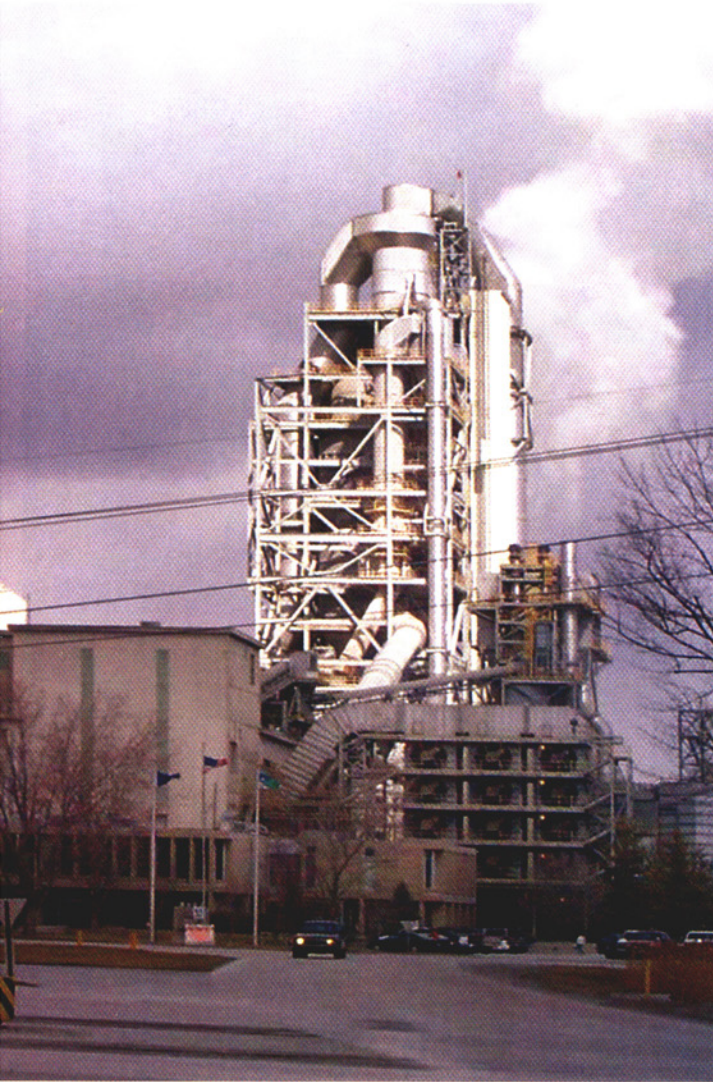
Greencastle cement plant showing precalciner/preheater tower.
